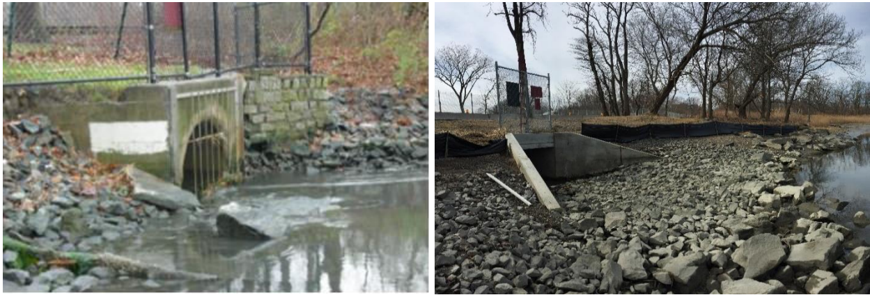
Figure 11. Example of an undersized culvert (left) in 2013 into Eastchester Bay and following replacement (right) in 2016 at Turtle Cove in Pelham Bay Park, Bronx.
