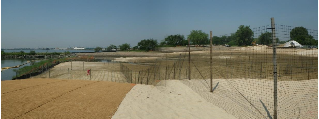
Figure 20: Example of coir webbing installed on upland slope at Soundview Park, Bronx.
