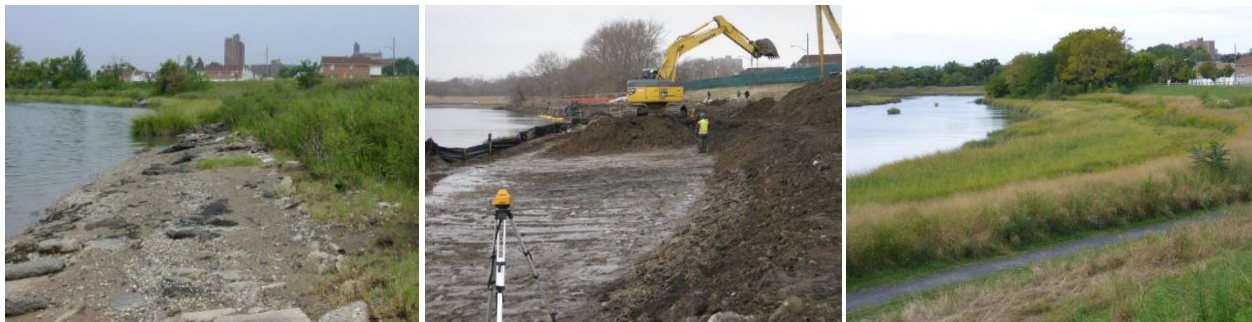
Figure 15. Salt marsh restoration involving over-excavation of fill and placement of clean substrate at Pugsley Creek in The Bronx, NY Images show the site before, ca. 2008 (left), during, ca. March 2011 (middle), and after restoration, ca. September 2015 (right).
