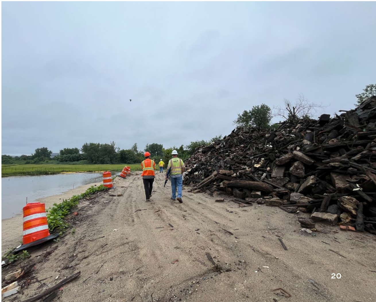
Construction debris for removal in Idlewild Park
